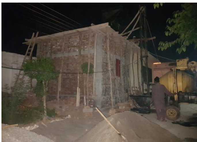
DRC Roof Slab Work
