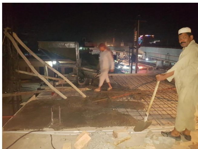
DRC Roof Slab Work
