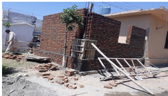
Brick Masonry work at DRC hall
